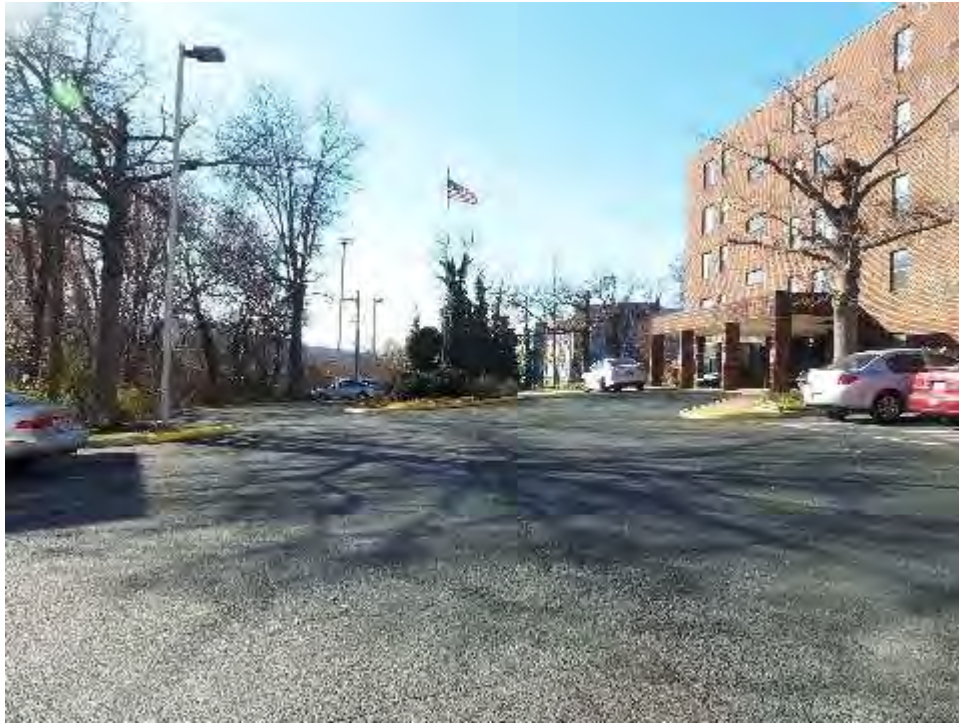
View of Parking
